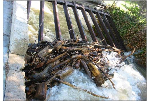
Trash racks are necessary to catch stream debris before it can cause serious damage during high flows, such as clogging culverts or snagging on bridge crossings. Help keep yard waste out of the stream in the first place!
