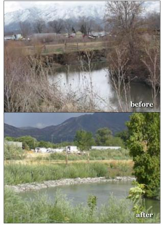
Vertically eroding banks are clearly visible in the "before" picture at one of seven Jordan River sites to receive stimulus funds for restoration. Bank stabilization included regrading the banks, placing a rock layer to protect the base (toe) of the slope, and revegetating with native plants.
